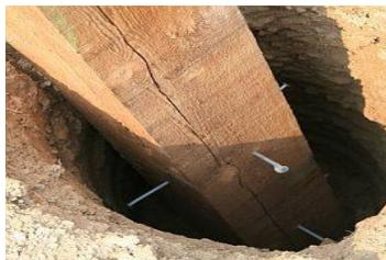
If additional posts are required, we recommend the use of a minimum 4 inch, schedule 40 steel pipe or 6inch x 6inch pressure treated wood. Your local timber supplier can assist you in selection. Post lengths should be taken into account with the proposed height of the sail plus the depth of your footings. Footing depth should be a minimum of 36 inches deep and 30inches square. For example, if your post height is higher than 8 feet, we recommend a hole depth 40% of the height above ground.
