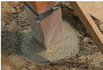
Mix concrete in line with the package instructions. These will be labeled clearly on the packet. Your supplier will be able to give you any special advice you may require for your own conditions. Pour concrete to the top of the holes ensuring it is packed well. Ensure the concrete surface is sloping away from the posts to assist water drainage. Allow poles to set in concrete for a minimum of 48 hours. Brace if required.
